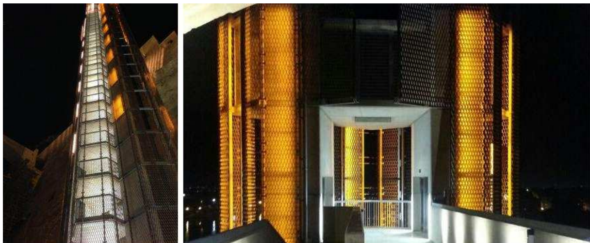
Figure 7 Launch of the Upper Barakka Lift
